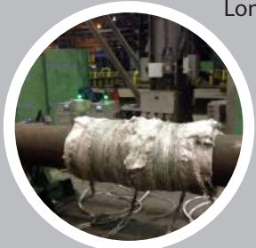
Circular Seam Heating
