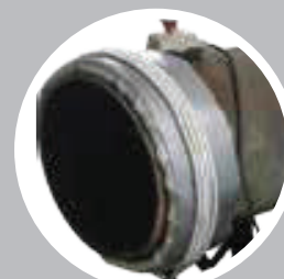
Circular Seam Heating
