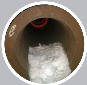
Long Seam Heating
