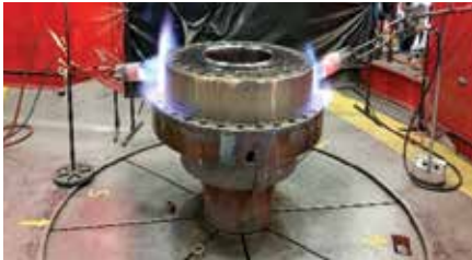
Heating with Gas Flame.
