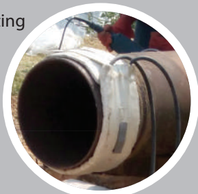
Pipe Line Heating
