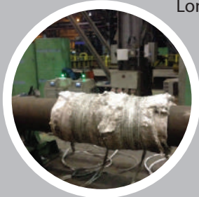
Circular Seam Heating
