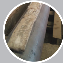
Long Seam Heating
